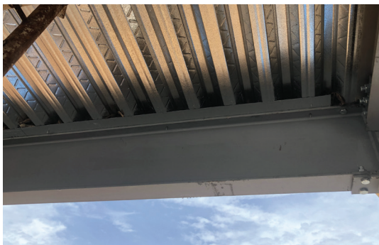
I-Beam Joint - Bottom View
