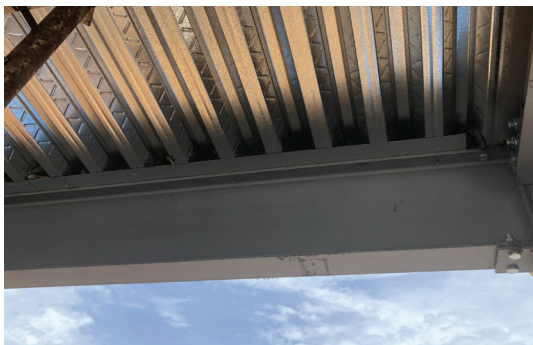
I-Beam Joint - Bottom View
