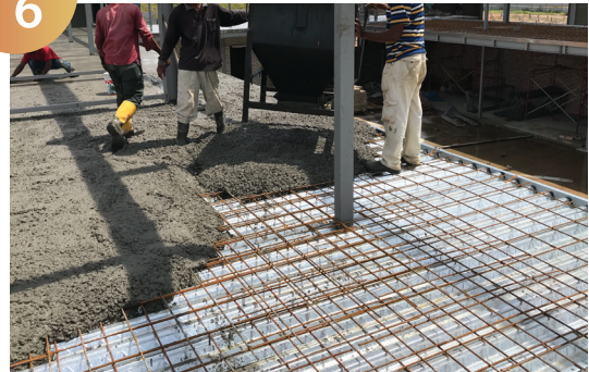
Pouring of Concrete Mixture
