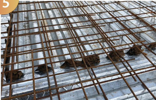
Sealing of Opening & Lapping
