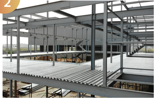
Laying of Floor Deck
