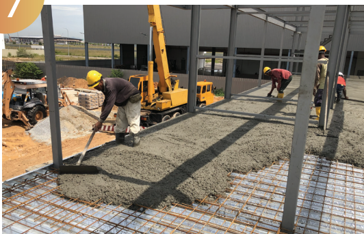
Concrete Mixture Levelling
