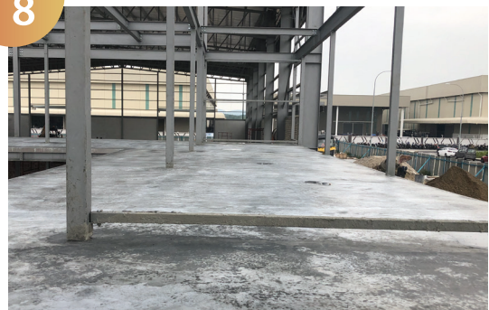
Concrete Mixture Curing
