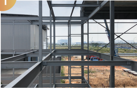
Installation of structure
